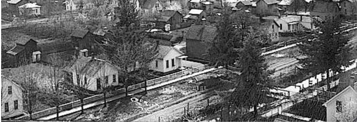
Figure 15: View of Millrace from Willamette Valley Milling Company
